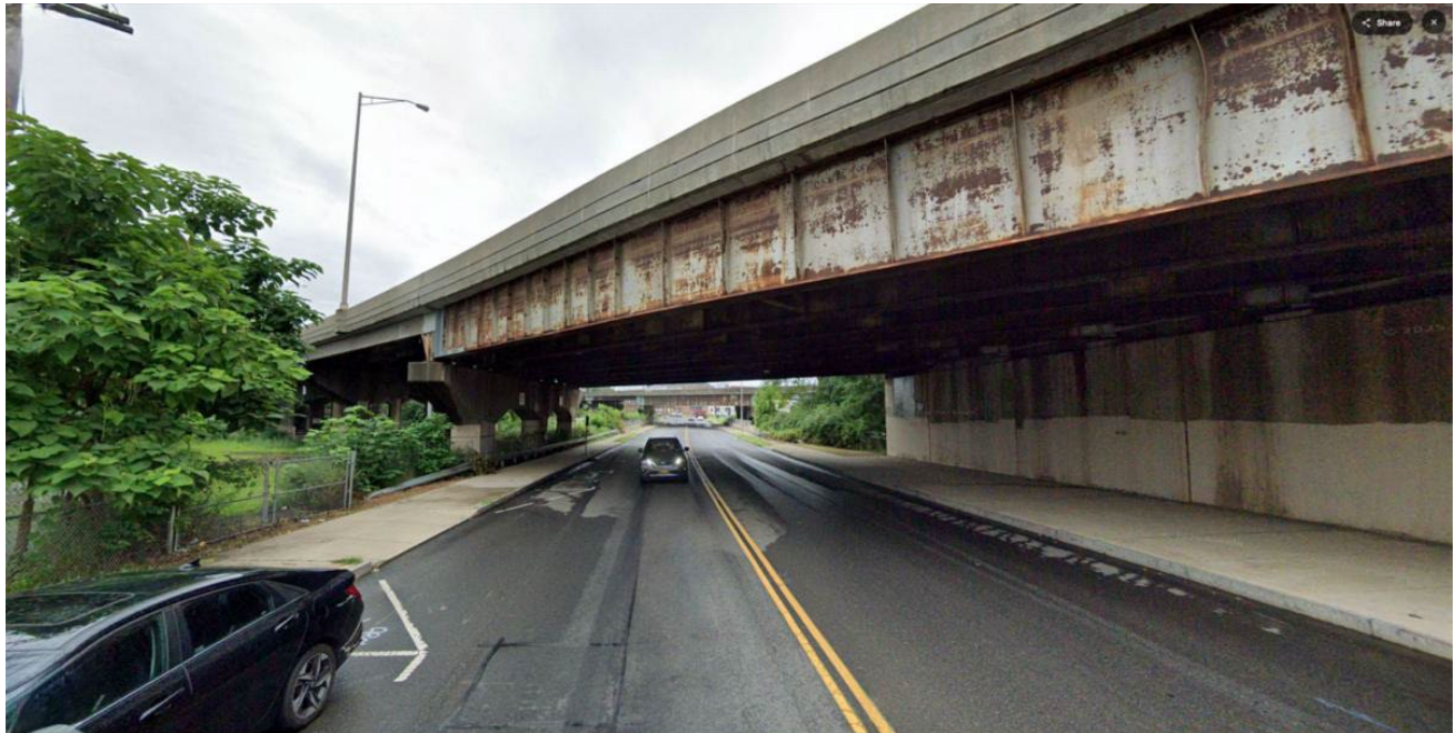
The perfect engineering-designed intersection of roadways carved out of what once were vibrant, if impoverished, neighborhoods within the city. The gash decapitates the remaining neighborhood on the “other side.” Photo courtesy of Robert Orr.
