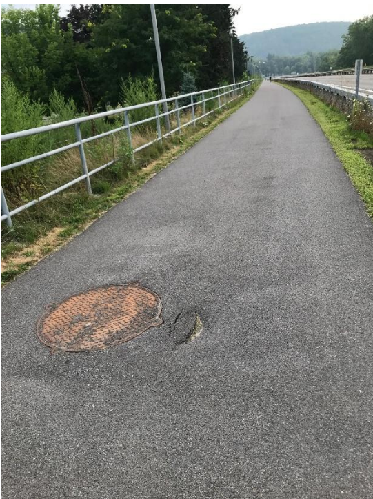
Photo 3: Cracking/Depression at Hallam Street to MacArthur Park (View 3)
