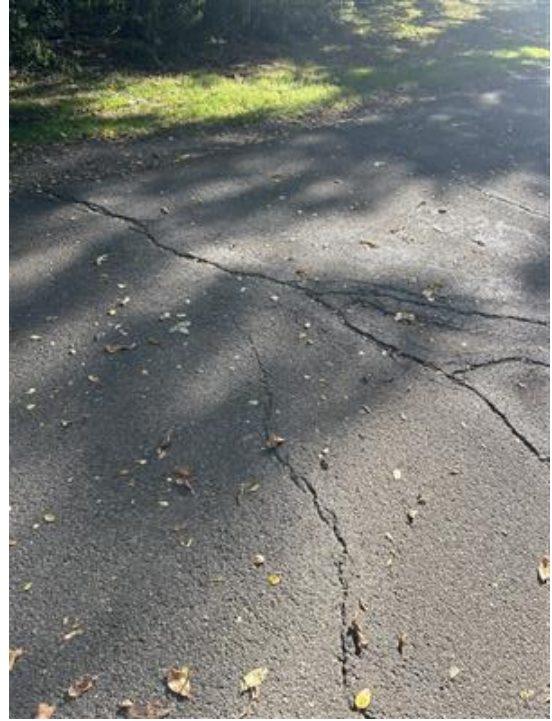
Photo 31: Cracking at Twin Orchards Park Adjacent
