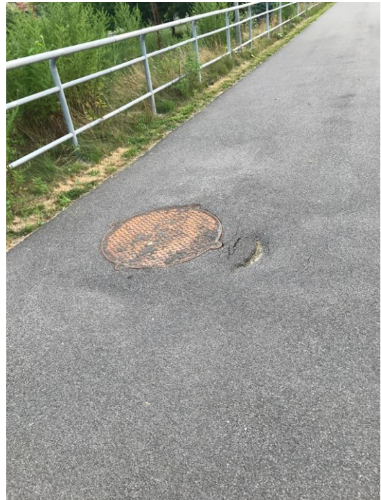
Photo 2: Cracking/Depression at Hallam Street to MacArthur Park (View 2)
