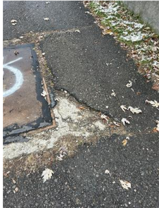
Photo 14: Cracking at UE Tennis Courts to Endicott Village Water Department
