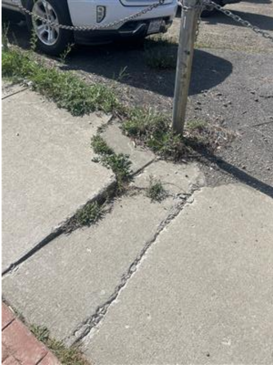
Photo 10: Cracking and Sinking at E Clinton Street to Eldredge
