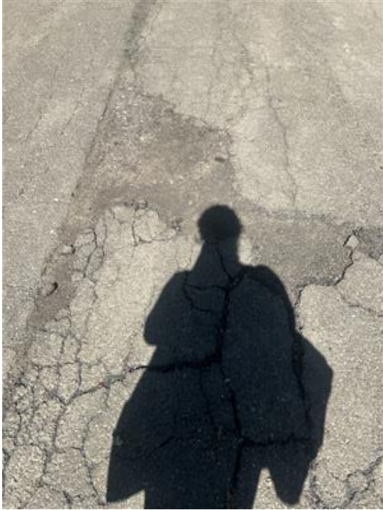
Photo 29: Raveling at Southern Inner Path
