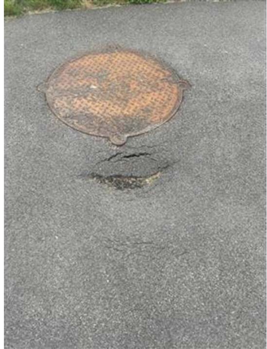
Photo 6. Cracking/Depression at Hallam Street to MacArthur Park
