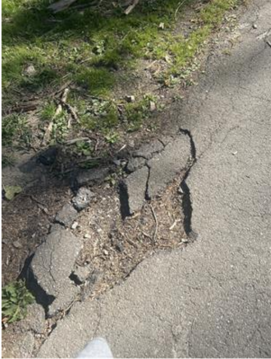
Photo 19: Cracking at Otsiningo Riverwalk
