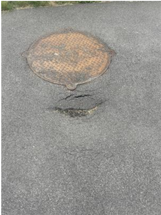
Photo 1: Cracking/Depression at Hallam Street to MacArthur Park (View 1)
