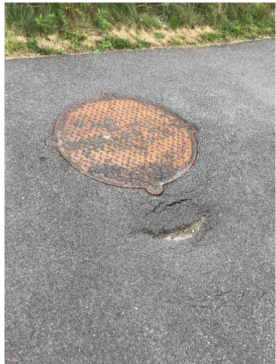
Photo 4: Cracking/Depression at Hallam Street to MacArthur Park (View 4)
