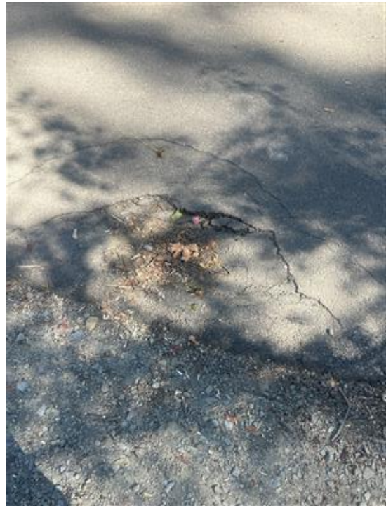
Photo 18: Cracking and Depression at Otsiningo Park Loop East
