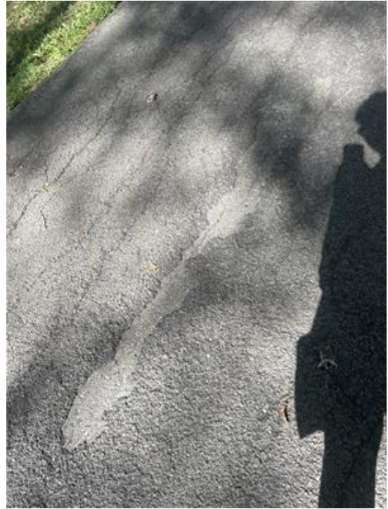
Photo 22. Asphalt Loss at Southern Loop Segment
