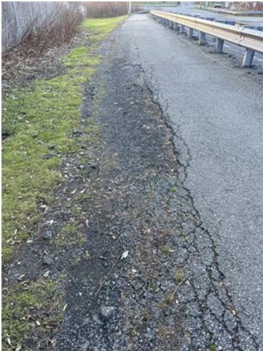
Photo 32: Raveling at Stroehmann Bakeries
