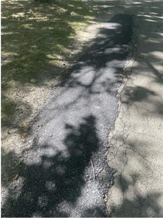
Photo 21. Asphalt Patch at Center Path/Western Loop Segment
