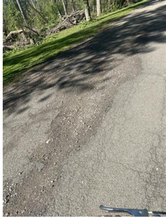
Photo 20: Cracking and Raveling at Northern Upper Front Street
