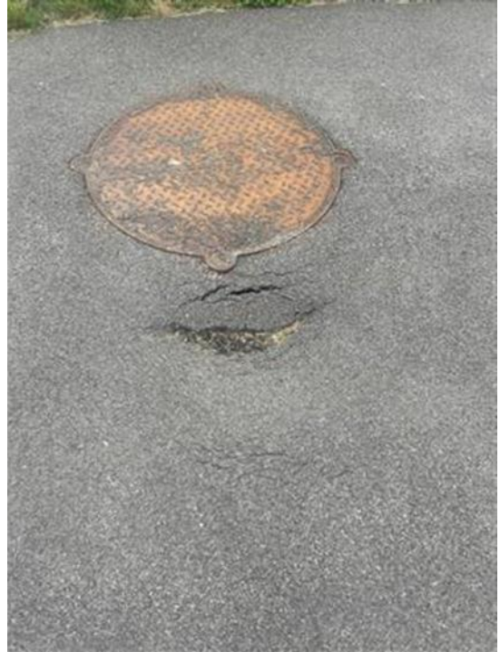
Photo 6. Cracking/Depression at Hallam Street to MacArthur Park
