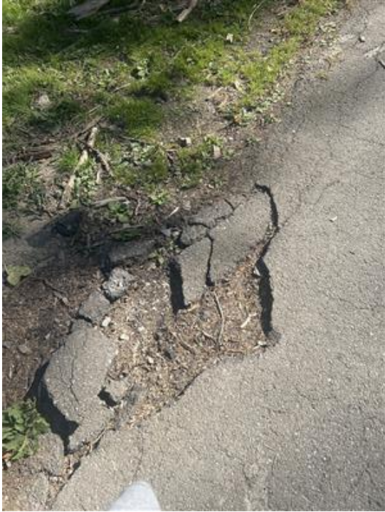
Photo 19: Cracking at Otsiningo Riverwalk
