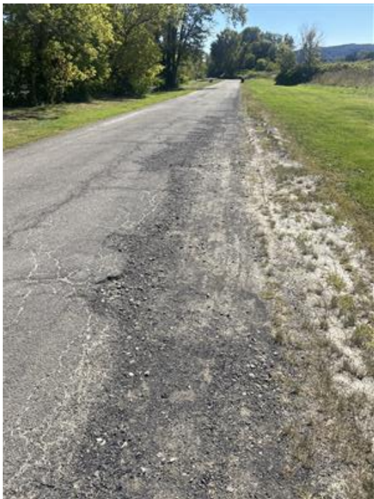
Photo 21: Cracking and Raveling at Northern Upper Front Street
