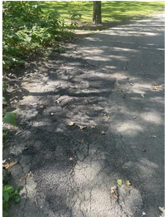
Photo 26: Raveling at Southern Loop Segment
