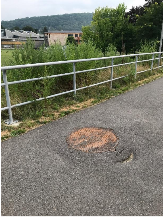
Photo 5. Cracking/Depression at Hallam Street to MacArthur Park (View 5)
