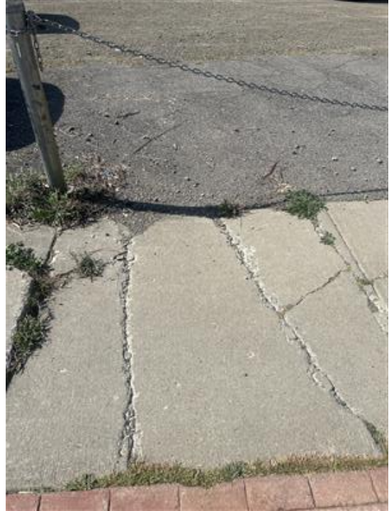
Photo 8. Sidewalk Cracking at E Clinton Street to Eldredge
