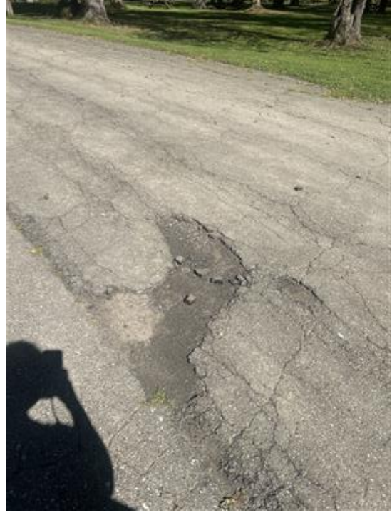
Photo 28: Raveling at Southern Inner Path
