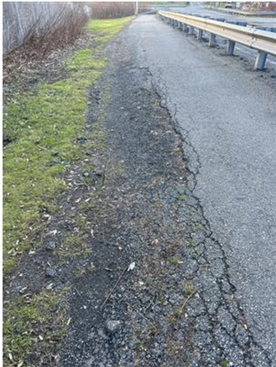
Photo 32: Raveling at Stroehmann Bakeries
