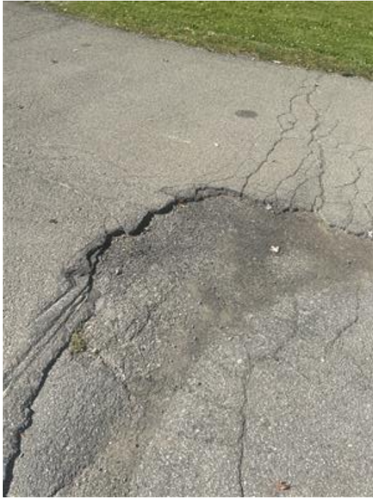
Photo 15: Cracking and Depression at Otsiningo Park/Route 11 Connection
