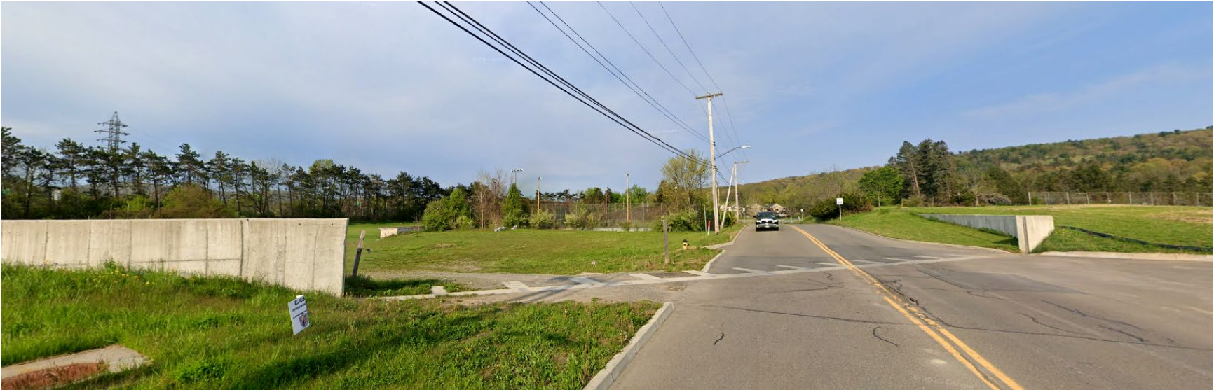
Flood gate east of Barton Avenue, part of the Fairmont Park levee system.
