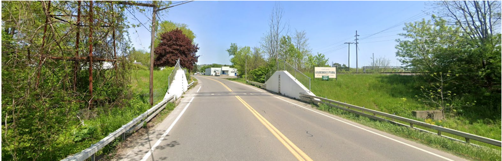
Flood gate west of Poplar Street, part of the Fairmont Park levee system.
