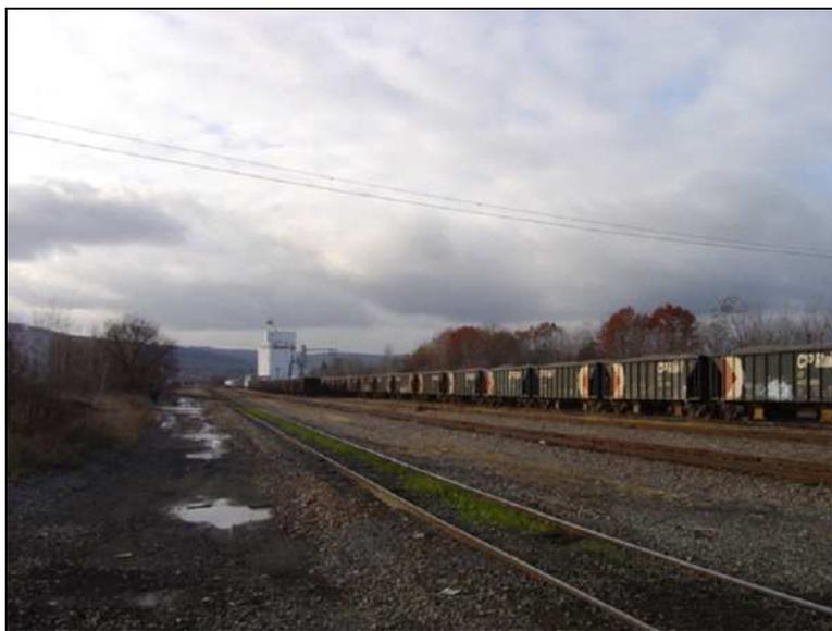
The NYSW Binghamton Yard is located in central Binghamton between Chenango Street and Brandywine Avenue. NYSW can transload freight from up to 15 railcars at the facility via a loading dock. NYSW primarily transloads iron and steel scrap at the yard. In addition, both NYSW and CNYK exchange cars with NS at the Binghamton Yard.
