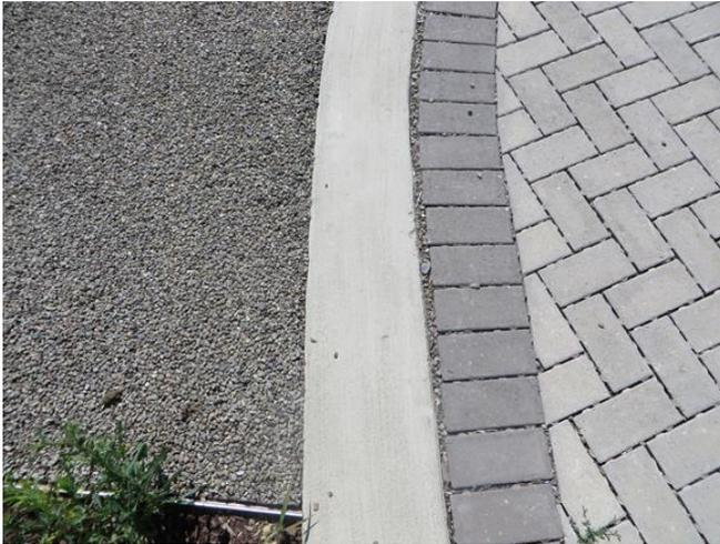
Figure 16: Permeable concrete and permeable pavers, McArthur School, Binghamton
