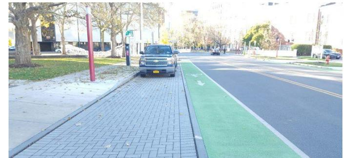
Figure 18: Pervious On-street Parking, Syracuse (Source: Milwaukee Stormwater Plan)
