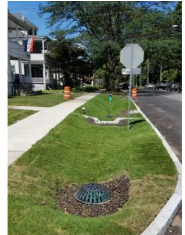
Figure 9: Streetside Bioswale, Syracuse (Source: Milwaukee Stormwater Plan)
