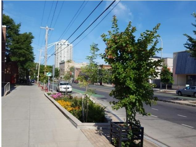
Figure 11: Stormwater Planter and Street Tree, Syracuse (Source: Milwaukee Stormwater Plan)
