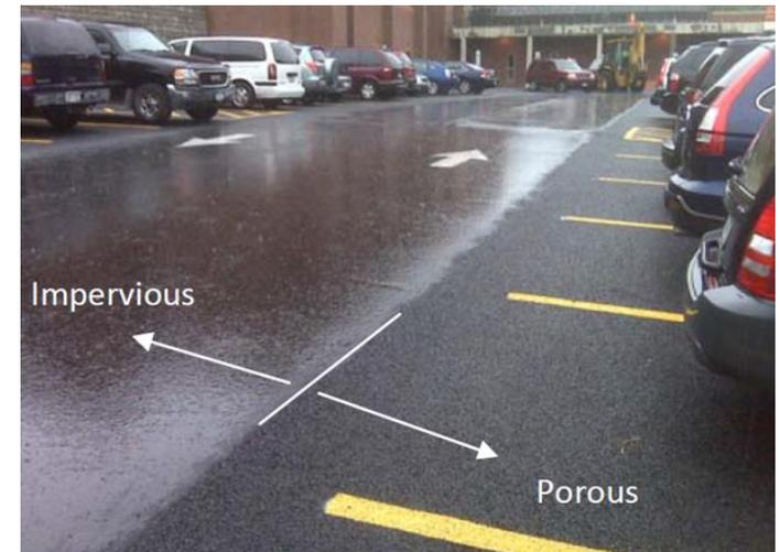
Figure 17: Permeable asphalt on-street parking during rain event, Syracuse (Source: Milwaukee Green Streets Stormwater Plan)
