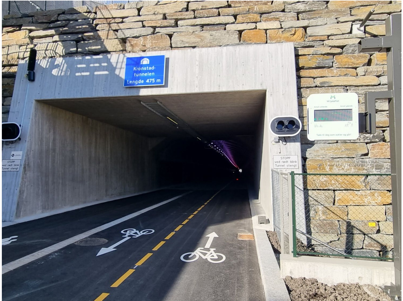
The new Kronstad tunnel joins Bergen's burgeoning bike infrastructure network. Photo: Einar J. Grieg/City of Bergen
