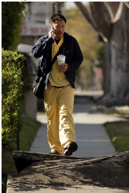
An LA resident navigates a sidewalk in dire need of repair. Photographer: Rick Loomis/Los Angeles Times via Getty Images
