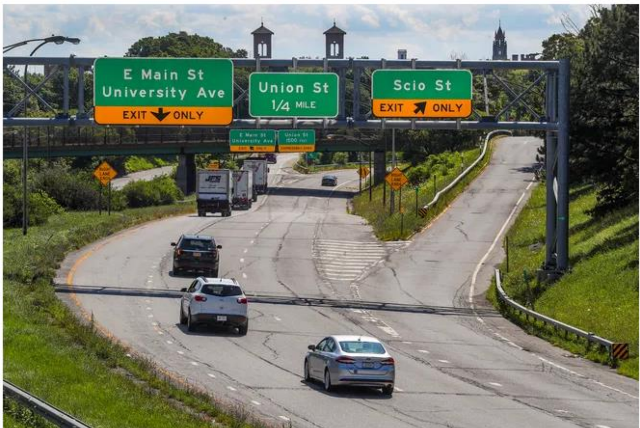
A view of the Inner Loop where major construction will have an impact on that neighborhood. JAMIE GERMANO/ROCHESTER DEMOCRAT AND CHRONICLE
