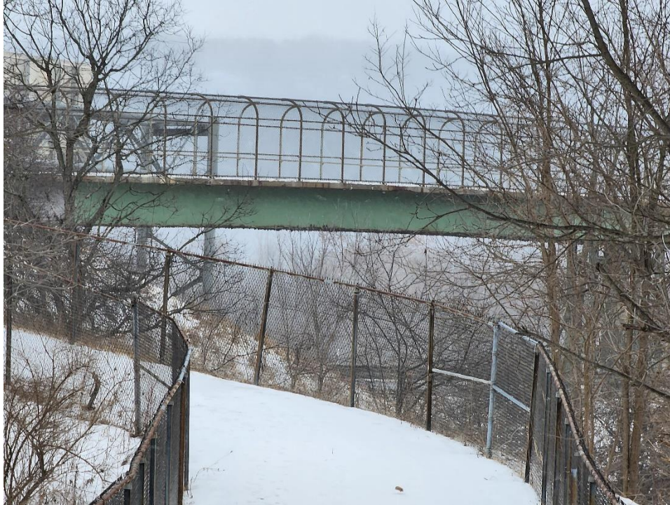
A pedestrian bridge in the town of Dickinson on February 3, 2023. (Photo: Bob Joseph/WNBF News)
