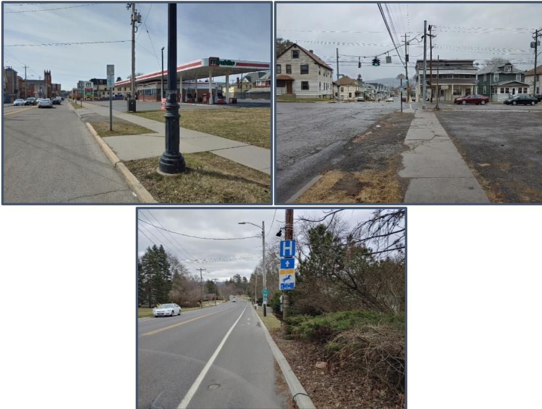
Figure 4 - Examples of Sidewalk Conditions Classified in the Inventory as 'Good' (top-left), 'Poor' (top-right), and 'Missing' (bottom).
